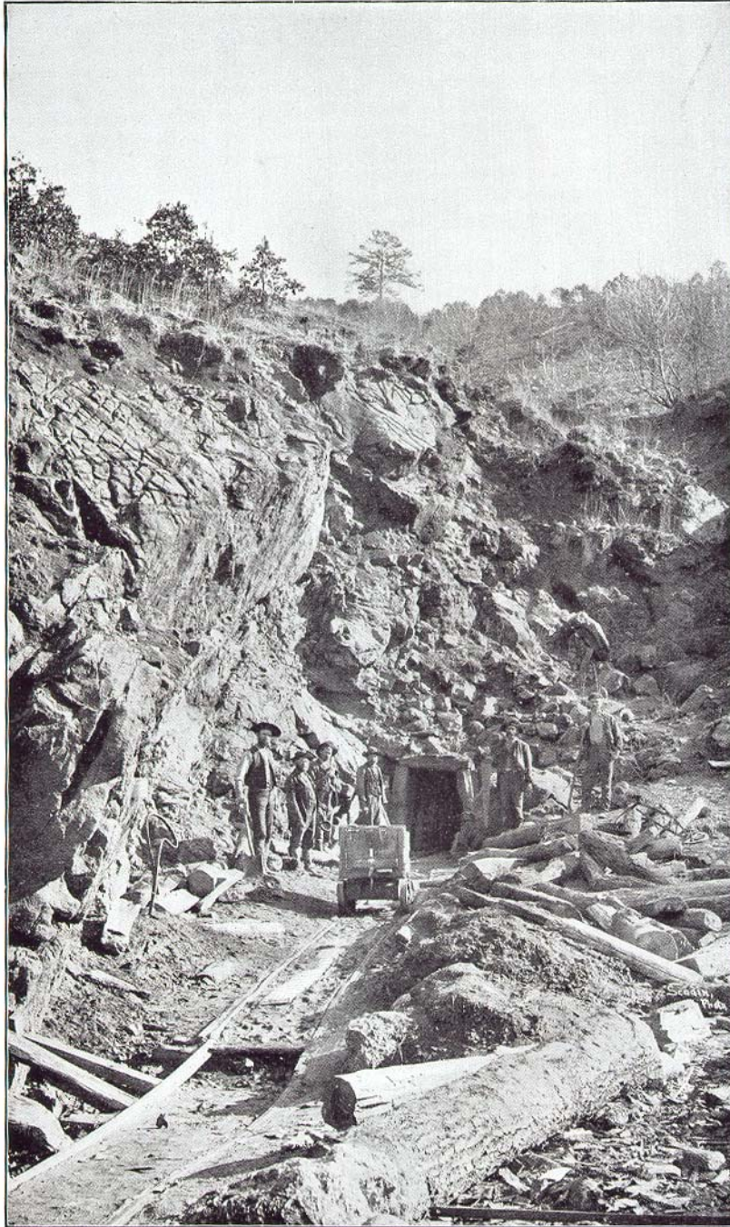
ENTRANCE TO TUNNEL ON BIG VEIN, BETWEEN PERIDOTITE AND GNEISS, CORUNDUM HILL, MACON COUNTY, N. C.
